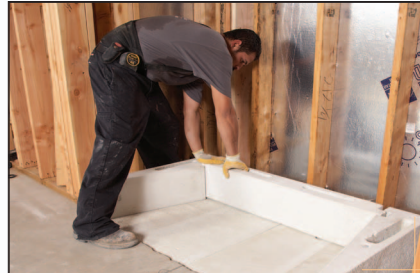
1. Installing base and first course
