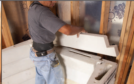
2. Starting the smoke chamber
