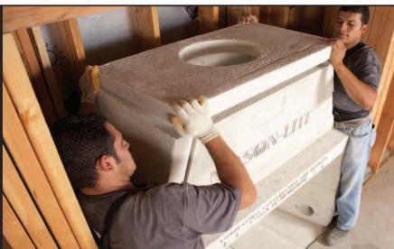
4. Finishing with the dome top
