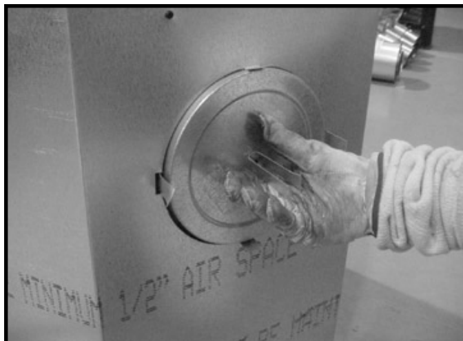
Figure 6.8 (Generic Fireplace Shown) Fold the center parts of the retaining band out and use to remove the seal cap.
