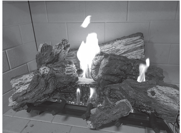
Figure 5.13 - Correct Appearance of Rear Flames
