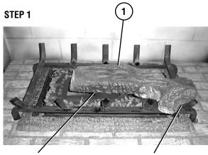
Position Groove At The Bottom Of Log (1) Over The Burner Log Support Bracket Position The Groove At The Bottom Of Log (1) Over The Grate And Slide It Forward Against The Grate Here
