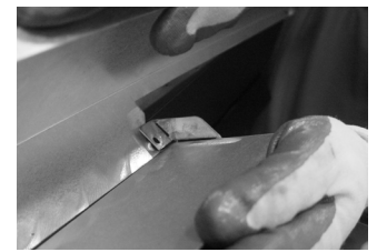
Step 1: Carefully bend up the two (2) tabs on the heat shield at a 90° angle from each opposite joint and then the foot of the Standoff at approximately a 45° angle.
