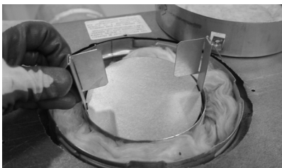
Step 4: Make sure insulation disc is still in the round cover. Remove the flue plug from the top flue.
