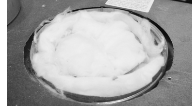
Step 3: Remove insulation from inside flue pipe.
