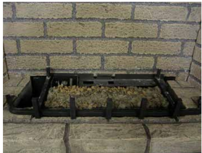
Figure 39 - Placement of Rock Wool on Burner
