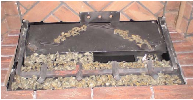
Burner Grate Assembly
