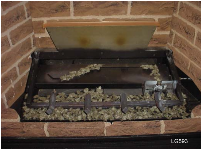
Burner Grate Assembly
