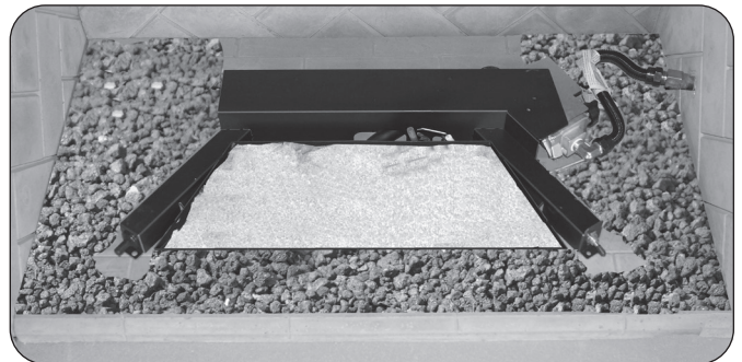
Fig. 20-3 Place sand/vermiculite
