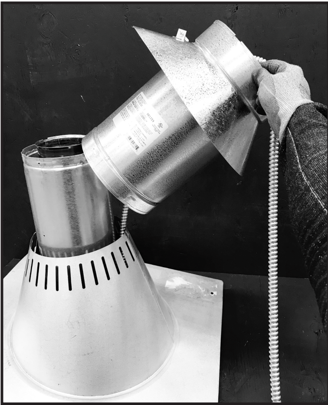
Figure 3.19 Route PVI Harness Through Flashing
