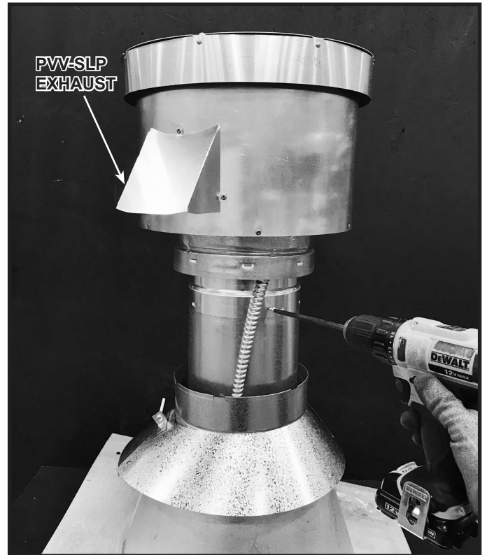
Figure 3.21 Attach PVV-SLP to SLP Pipe
