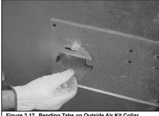
Figure 3.17 Bending Tabs on Outside Air Kit Collar
