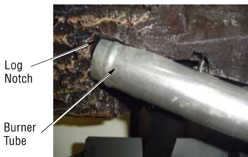
Figure 23A - Installing Back Left Log
