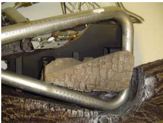
Figure 25A - Installing Charred Log Top View
