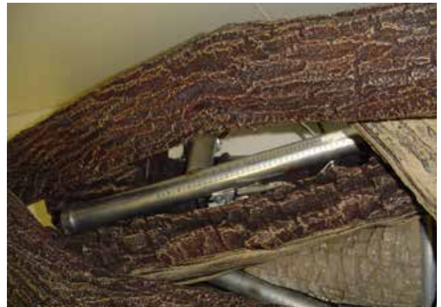
Figure 25A - Installing Back Top Log, Top View
