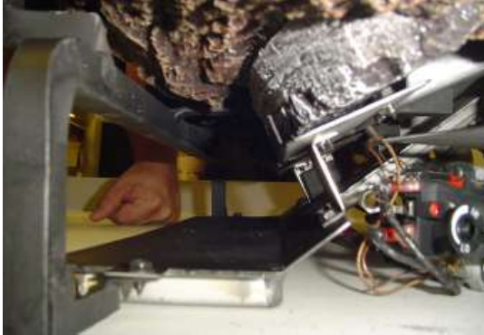
Figure 24C - Installing Right Front Log, Side View
