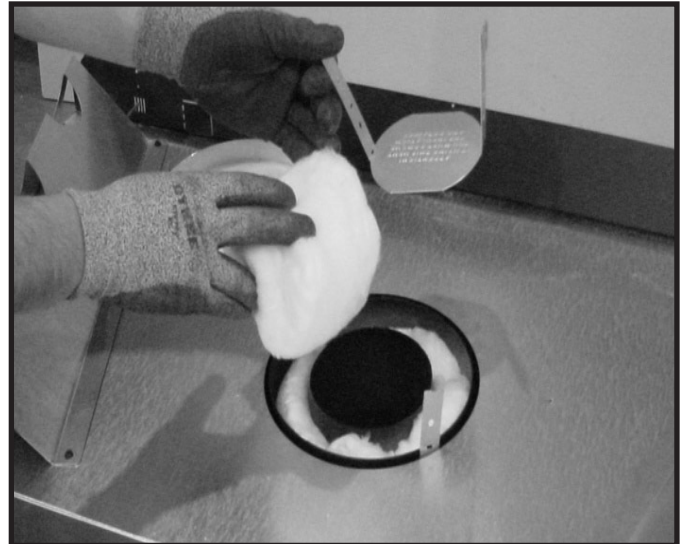
Figure 6.4 (Generic Fireplace Shown) Remove the insulation basket and white insulation from the center vent pipe.
