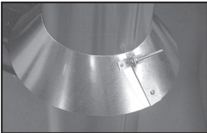
Figure 7.13 insert Bolt into Brackets
