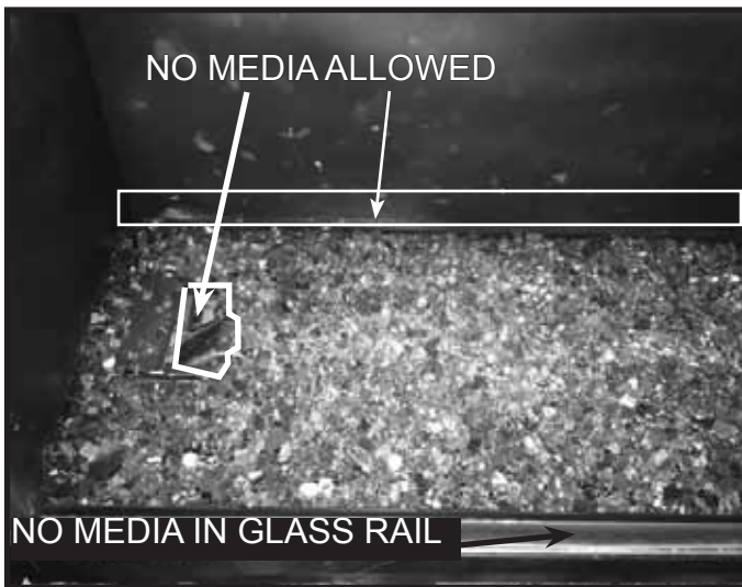
Figure 6. Media Installed
