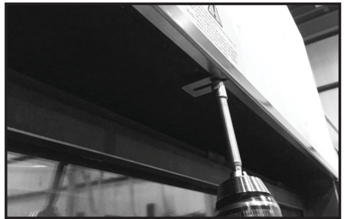
Figure 10.5. Install Trim Ring
