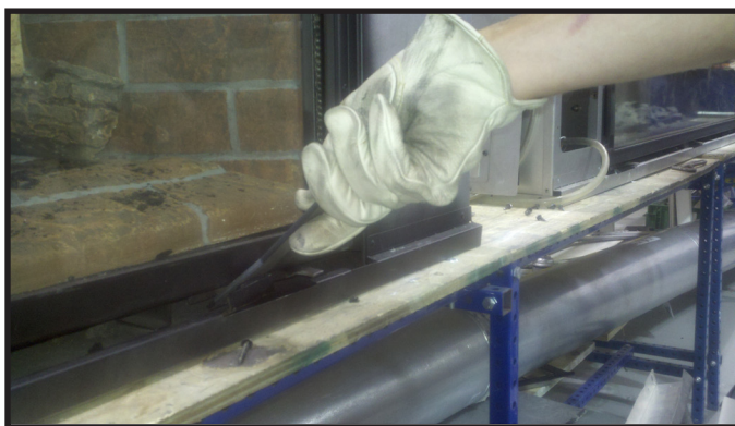
Figure 11.3. Inserting Glass Clip Tool
