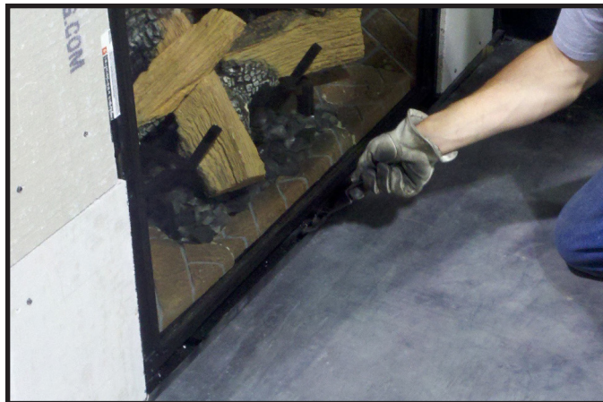
Figure 11.8. Securing Bottom Glass Clips
