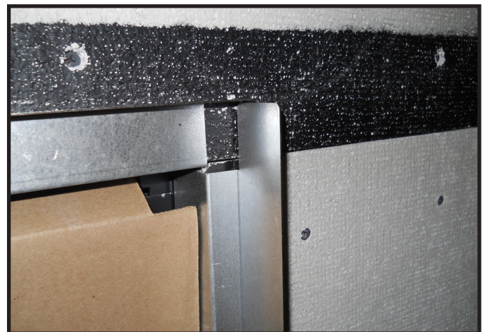
Figure 10.5 Finishing Template Bends
