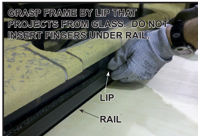
Figure 11.6. Installing Glass
