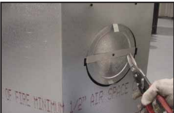
Figure 6.7 (Generic Fireplace Shown) Cut the metal retaining band and fold the sides out.
