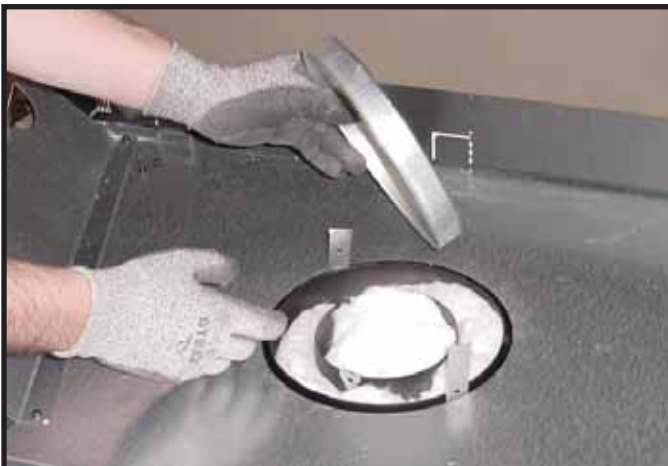
Figure 6.3 (Generic Fireplace Shown) Remove the seal cap.
