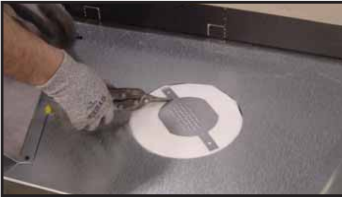
Figure 6.1 (Generic Fireplace Shown) Cut the seal cap strap across the rectangles next to the disk. For rear vent, skip this step.
