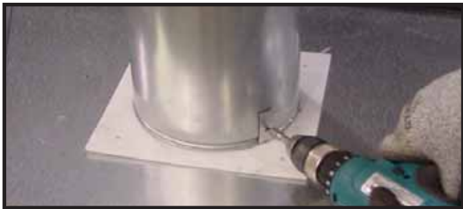
Figure 6.6 (Generic Fireplace Shown) To attach the first section of vent pipe, make sure to use the fiberglass gasket in the manual bag to seal between the first vent component and the outer fireplace wrap. Use 2 self tapping screws to secure the gasket to the outer wrap.
