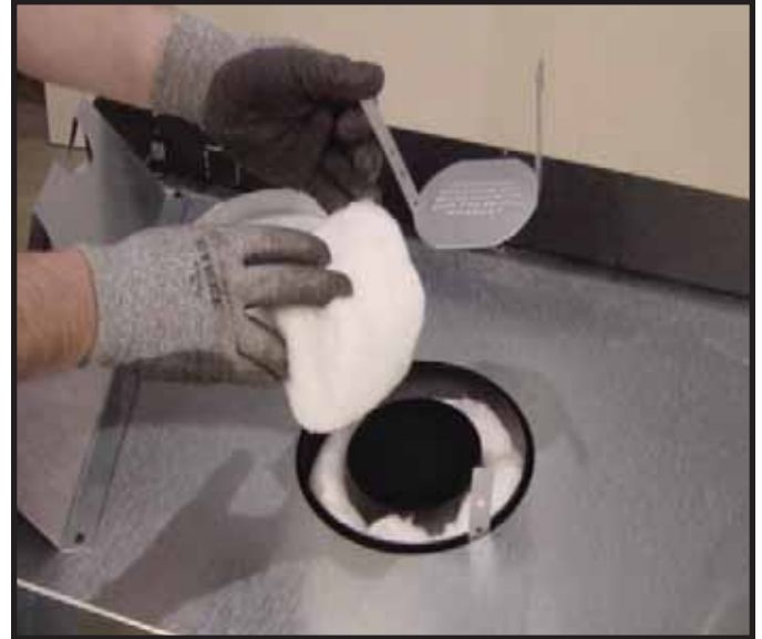
Figure 6.4 (Generic Fireplace Shown) Remove the insulation basket and white insulation from the center vent pipe.
