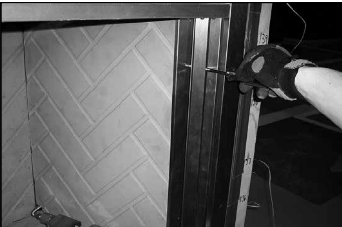
Figure 12.3 Loosen Refractory Retaining Strip
