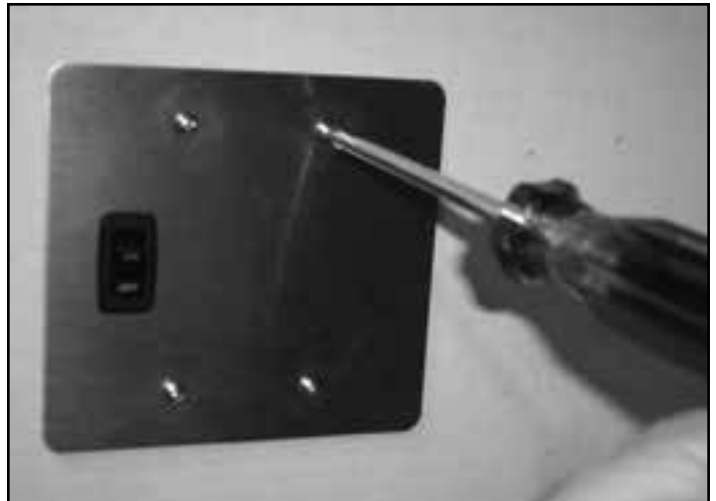
Figure 12.9 Switch Cover Plate
