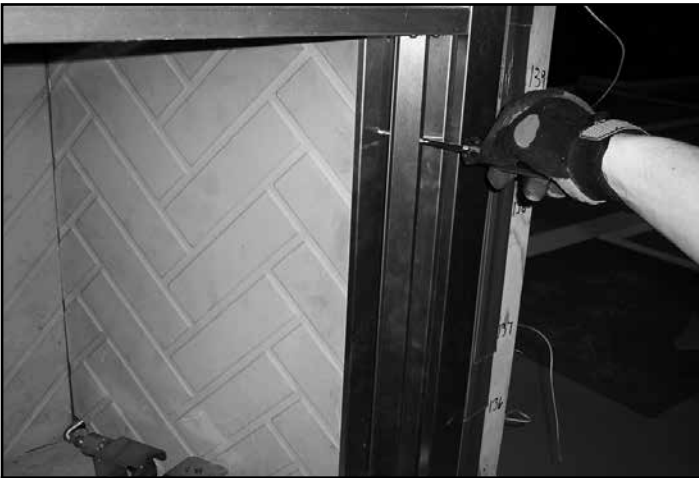
Figure 6.3 Loosen Refractory Retaining Strip
