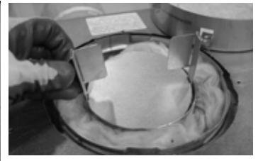
Step 4: Make sure insulation disc is still in the round cover. Remove the flue plug from the top flue.
