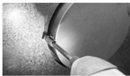
Step 6: Secure the round flue cover (provided) to the wrapper over the rear venting outlet. Use two (2) 3/4" long sheet metal screws
