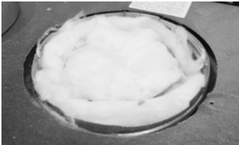
Step 3: Remove insulation from inside flue pipe.
