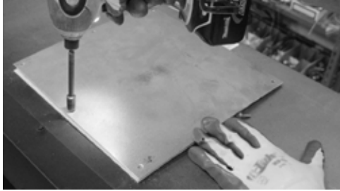
Step 1: Remove the eight (8) screws holding the top vent cover plate and gasket. Discard cover plate and reinstall screws.
