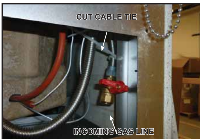
Figure 6.2 Connect Incoming Gas Line to Manual Shutoff Valve
