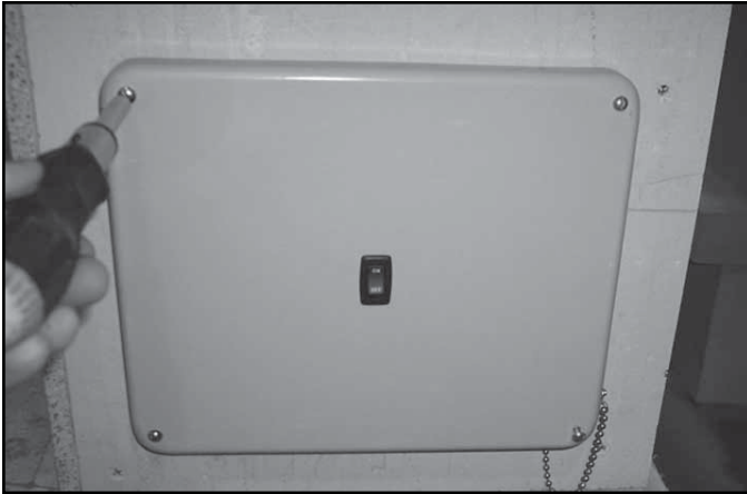
Figure 5.1 Remove Control Cover
