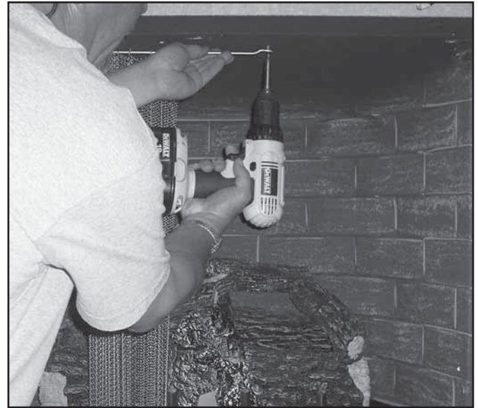
Figure 8.17 Fasten Screen Rod to Firebox Top
