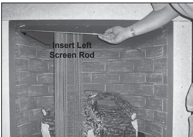
Figure 8.16 Insert Screen Rod
